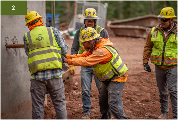
1. Constructing the wildlife crossings required excavating an area under the interstate. These arch-shaped bypasses will accommodate creatures of all sizes to safely pass through. 2. The construction crew installs and secures a structural anchor, working together to keep the project moving forward.
