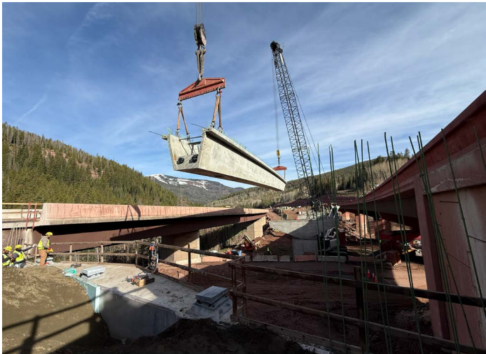
Crew members place a tub girder for the new bridge. Its tub-shaped design provides the strength needed to resist bending and twisting forces, helping support the bridge under years of heavy traffic.
