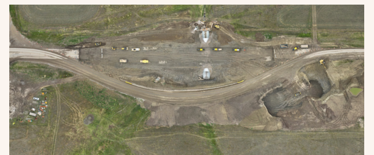
July – Backfill pipe and reconstruct roadway
