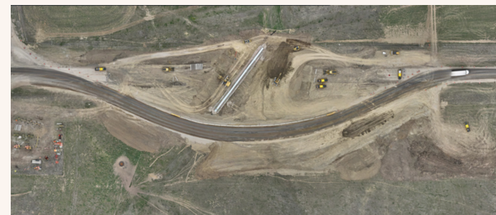
April – Remove existing roadway and timber bridge; install 60" drainage
