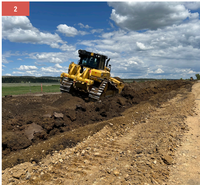
1. Kiewit crews and local landowners turned a campfire conversation into a pig roast with a band and about 50 people. 2. Crews perform earthwork along the corridor as part of bridge replacements and roadway improvements across the project.
