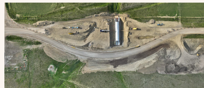
June – Assemble 20-foot-diameter multiplate pipe
