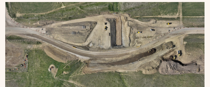
May – Excavate for 20-foot-diameter steel multiplate pipe
