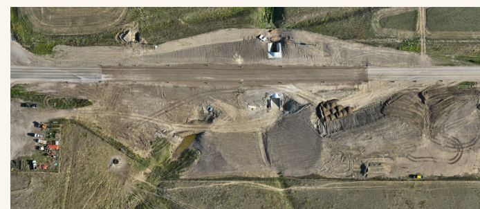
August – Complete grading; remove detour; place road base and drainage headwalls
