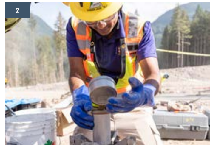
1. Structure crews use jump forms to construct the cast-in-place walls that form the barrier's centre slot. The slot allows the river and small-scale debris to pass through while helping protect downstream communities during major debris flow events. 2. Field Engineer Karan Jain receives training on concrete quality control testing. Two years later, Jain serves as project engineer, one of many team members who grew into expanded roles over the life of the project.
