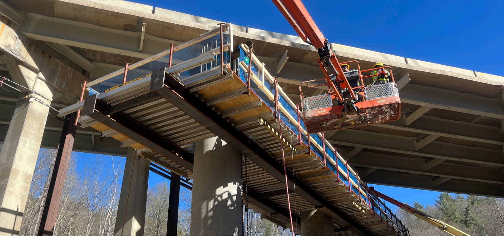
Kiewit employees erect a soffit for one of the new caps on the substructure of Bridge 142 over the Pigeon River. The three-span bridge is about 50 feet tall, 364 feet long and 81 feet wide. The substructure is designed to hold 63-inch Florida I-beams that weigh up to 71 tons.
