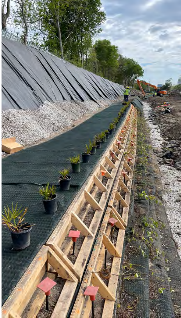
Pictured left: Vegetation cleared from the site was reused in many applications, including to build in-stream structures, as shown here. Pictured above: The vegetated reinforced stabilized slope (VRSS), a key element of the project's design, was built up in part using repurposed organic materials from site clearing.
